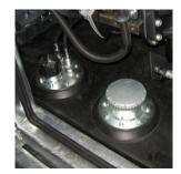
**Fuel tank** Fully bunded, corrosion-free, 300 liter, high-density polyethylene (HDPE) fuel tank, located in base of canopy.
